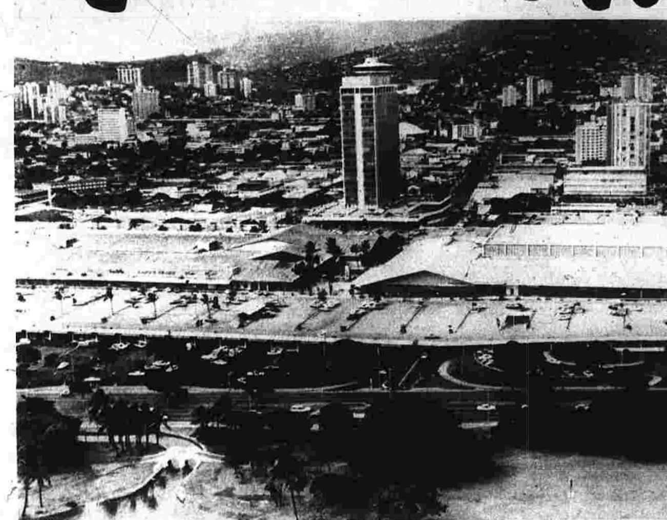
A revolving restaurant tops the 25-story professional building at the Ala Moana shopping center in Honolulu, Hawaii.
